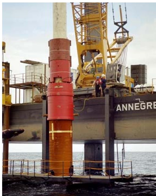
Figure 1: Hydraulic hammer on a pile of FINO1.
