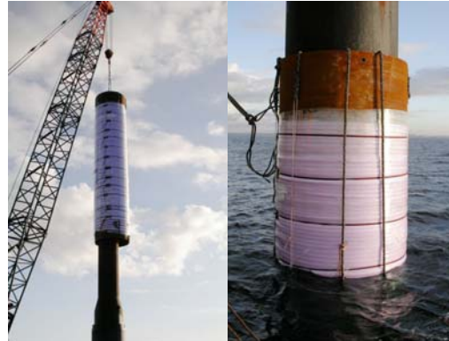
Fig. 9: Coated tube over a pile in the Baltic Sea.
